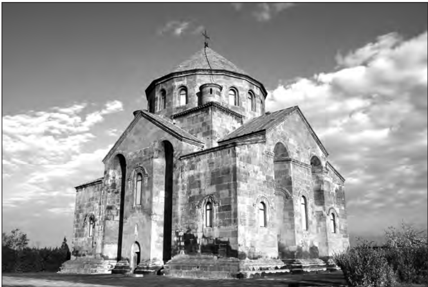
FIGURE 8.3. One of the oldest churches in Vagharshapat (Etchmiadzin), Armenia, Saint Hripsime Church, dates to the seventh century and features a raised dome and the shape of a cross at its base.
