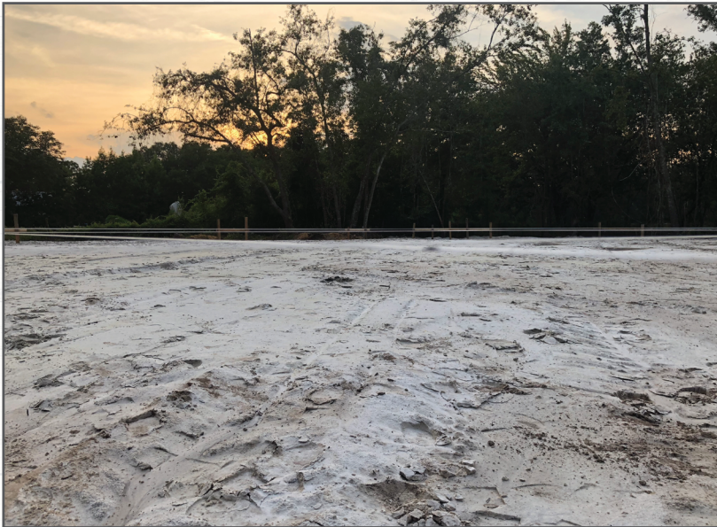
The land cleared and ready for building.
