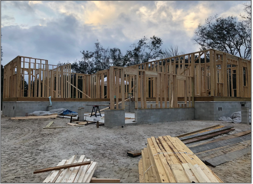
The house in the middle of framing.
